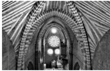
Vault of the nave © Michel Eisenhor
