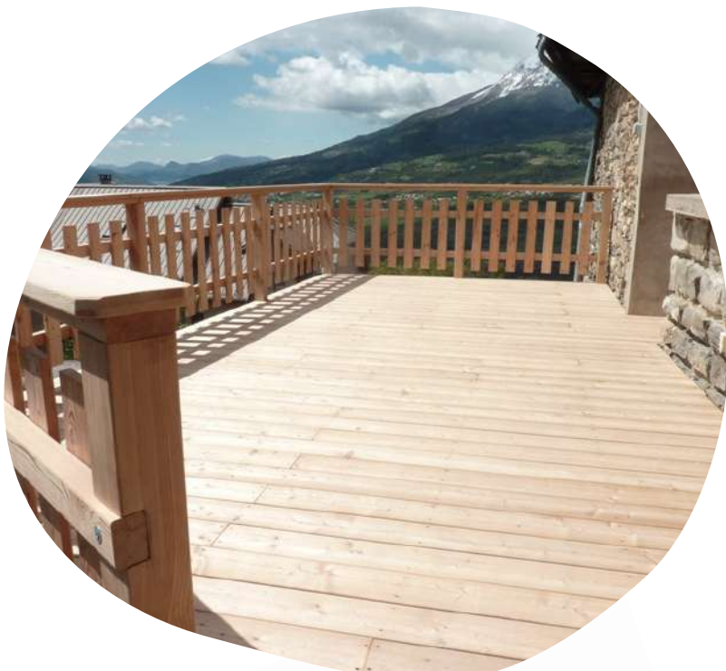
Terrasse bois – Source: eco 2 SCOP
